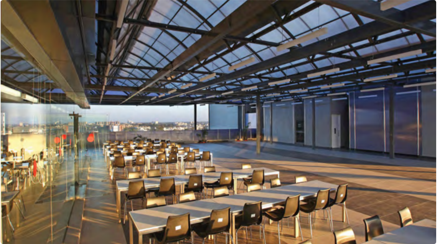
Mercedes Benz R&D Center, Bangalore, India | Architect: Atelier Architects Pvt Ltd – SMLXL Application: Skylight - 1500 sqm | SUNPAL® Type: Blue & Solar Control 18mm
