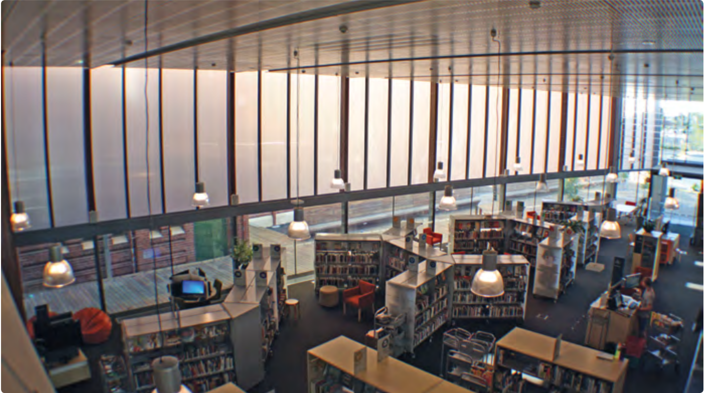
Williamstown Library, Victoria, Australia | Architect: Sally Draper Arch. | Application: Sidelight - 330 sqm | SUNPAL® Type: Solar Ice 18mm
