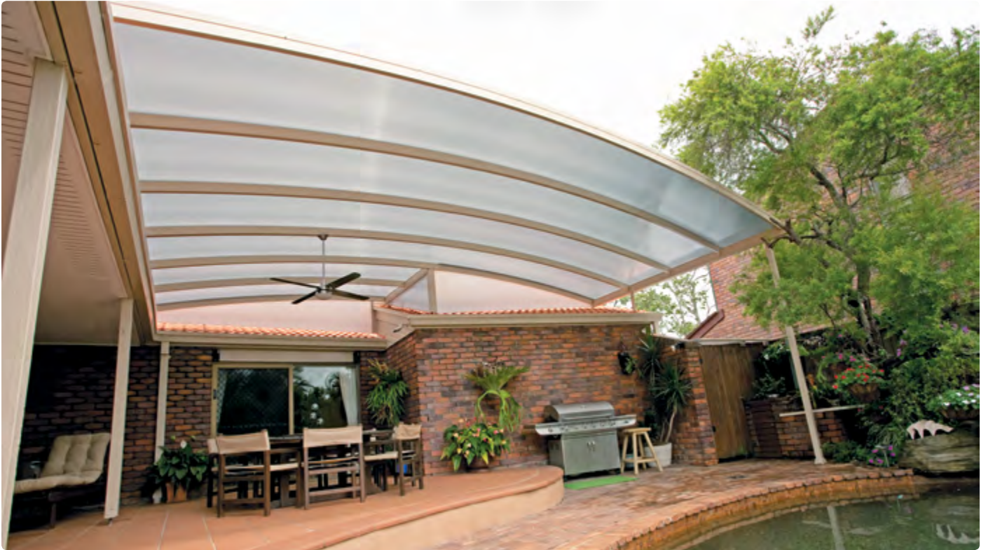
Private Residence, Brisbane, Australia | Application: Pergola | SUNPAL® - Solar Control 10mm
