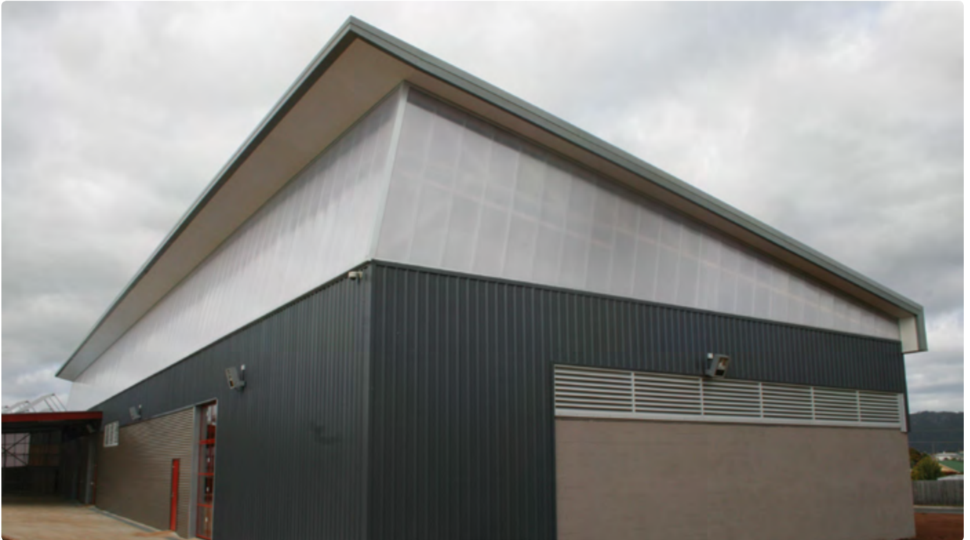
George Town Trade Centre Tasmania, Australia | Architect: Loop | Application: Sidelight | SUNPAL® Type: White Ice 10mm
