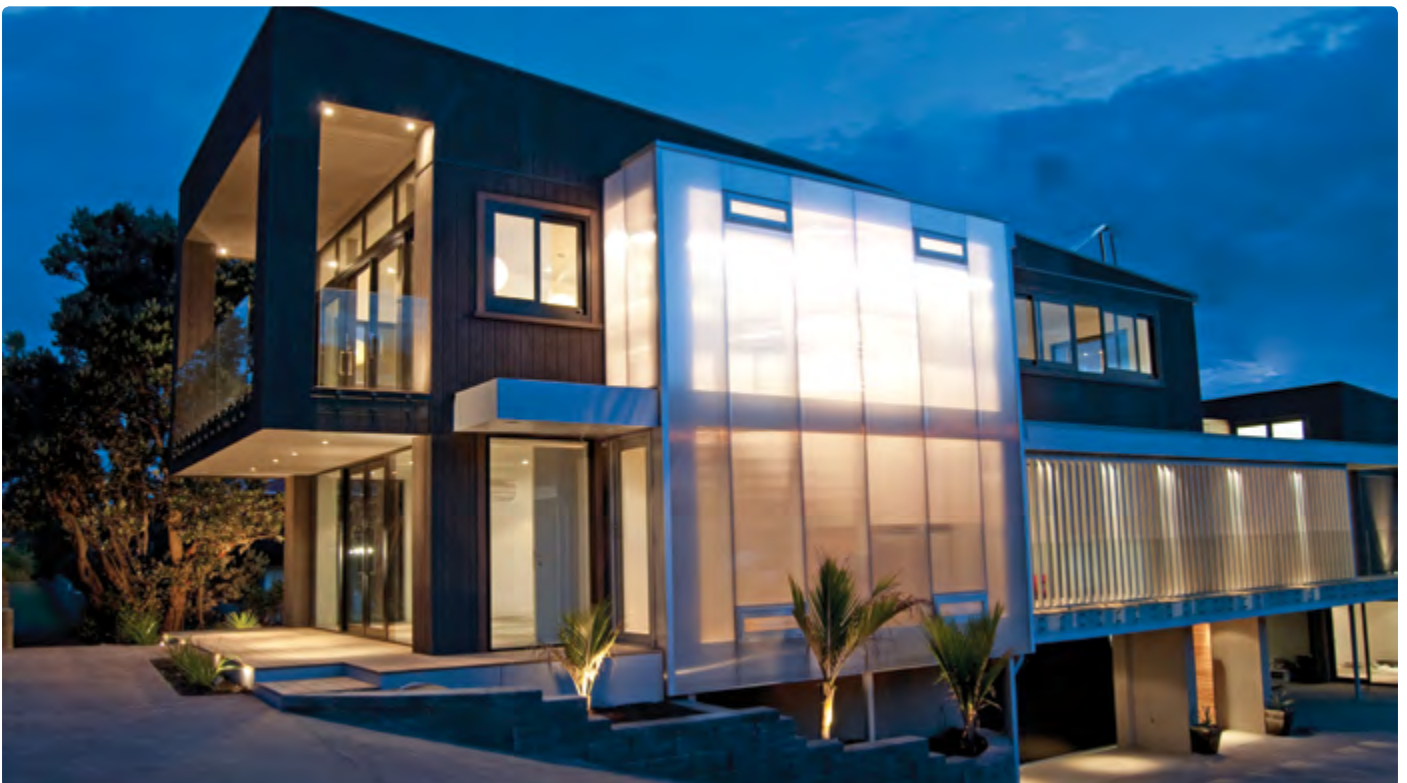
Private Residence, New Zealand | Application: Curtain Wall | SUNPAL® Type: Solar Ice 18mm
